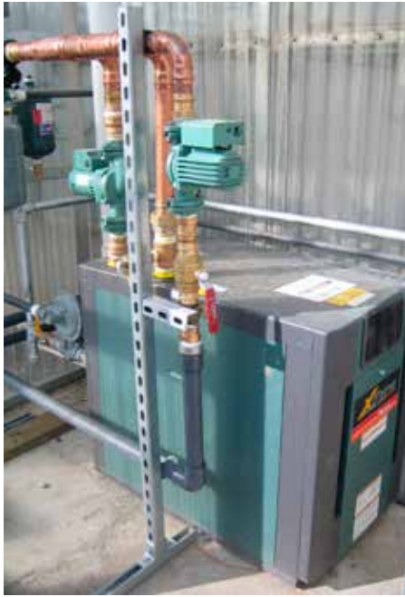
Left: Condensing boilers have a smaller footprint than cast iron boilers, and digital controls turn the boiler on when heat is truly needed. Right: The benchtop warm water tube heat focuses heat on seedlings and trays, saving energy on heating the entire space. PHOTOS COURTESY OF CHRIS GUNTERMANN
