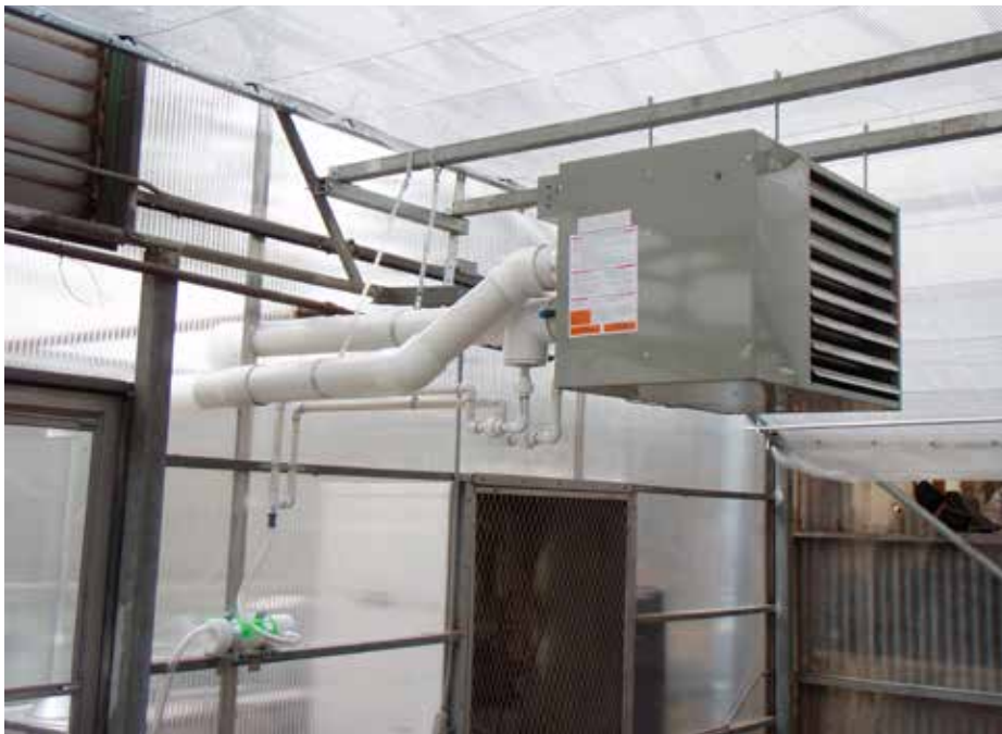
This condensing natural gas unit heater which shows the benefit of in-and-out venting using plain pvc pipe rather than stainless steel. It brings in outside air, burns it, then vents it back outside. The condensate line is shown, along with an acid neutralizer. PHOTOS COURTESY OF CHRIS GUNTERMANN
