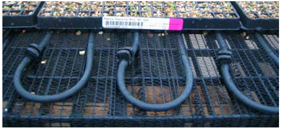
Left: Condensing boilers have a smaller footprint than cast iron boilers, and digital controls turn the boiler on when heat is truly needed. Right: The benchtop warm water tube heat focuses heat on seedlings and trays, saving energy on heating the entire space. PHOTOS COURTESY OF CHRIS GUNTERMANN
