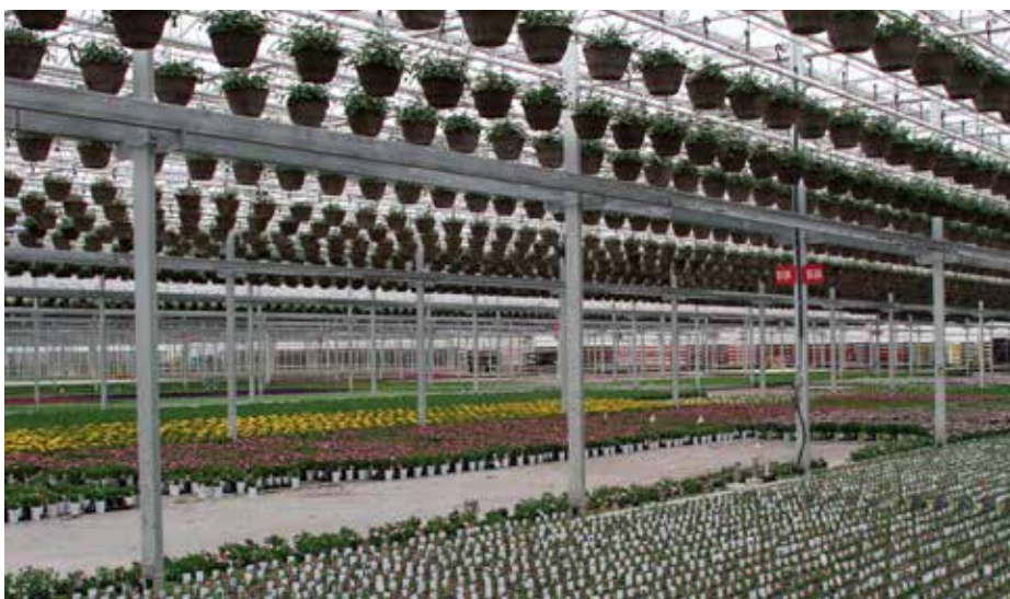
The new Smith Gardens greenhouse facility in Aurora, Oregon, uses frosted glass in order to eliminate shadows under baskets. PHOTO BY CURT KIPP
